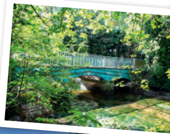
Ashen Road Iron Bridge.
